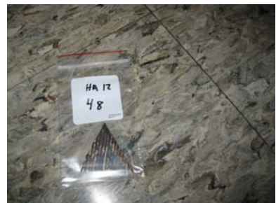
HA 12: Throughout building, 1x1 grey floor tile with specks
