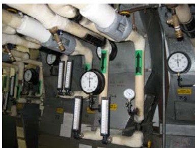
Photo 4: Room 206A, view of thermostats
