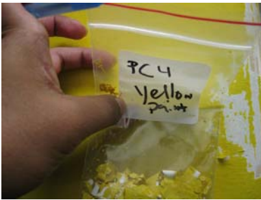
PC 4: 2 nd Floor male bathroom, yellow paint
