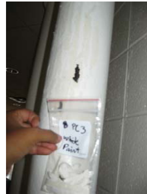
PC 3: Throughout building, white paint
