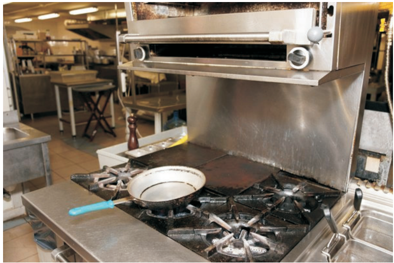
FIGURE 7. The blue insulated handle of this pan does not extend into the walkway. Is it a safety hazard?
