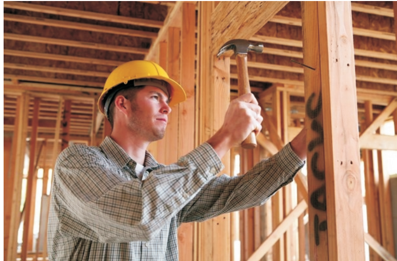
FIGURE 1. Carpenters are skilled volunteers who may be found at a Habitat for Humanity work site.
