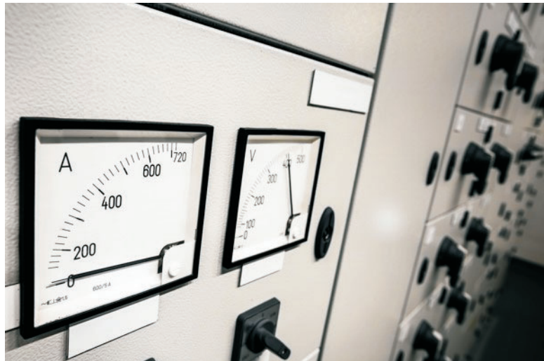
FIGURE 4. An ammeter measures the electric current in a circuit. A voltmeter measures electric potential—the difference in an electrical charge between two points in a circuit expressed in volts.
