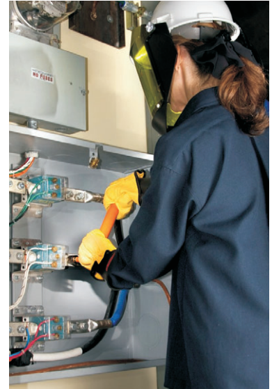
Electrician working on an energized panel.
