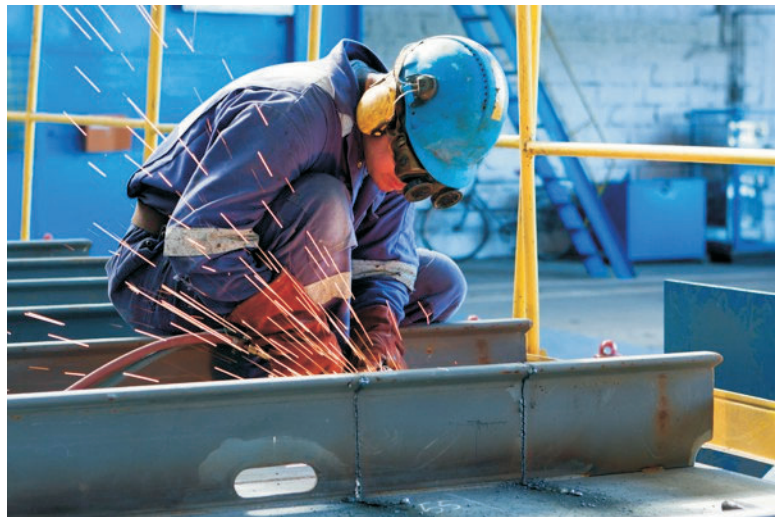
FIGURE 7. Field welding is a common practice. It is often necessary to complete repairs and intricate welds on site.
