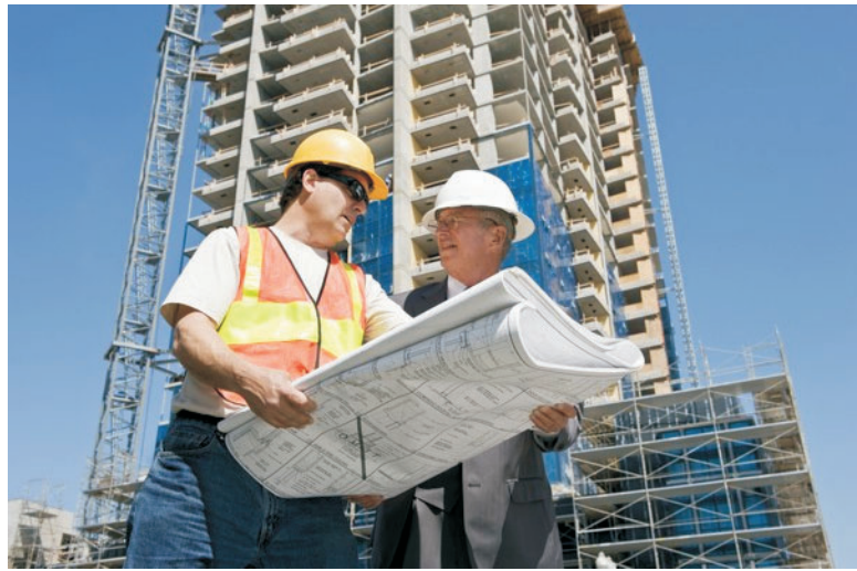
FIGURE 3. Developers and contractors—as shown in this image of a high-rise building under construction—may have different interests and long-term plans for the project. It is wise to include any key concerns—life cycle cost and risk assessment—in the project proposal and construction design brief.
