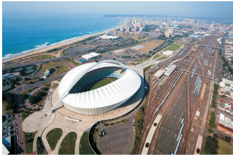
FIGURE 4. Many external factors can play a part in the success or failure of a construction project. External factors include weather conditions, such as buildings next to open water, or zoning and traffic patterns.
