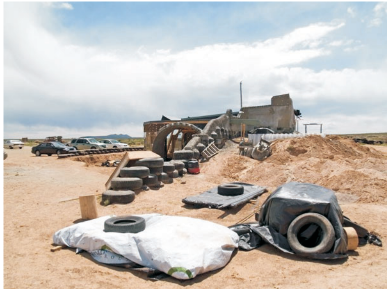
FIGURE 2. Earth is pounded into used tires to create the building material for Earthship homes.
