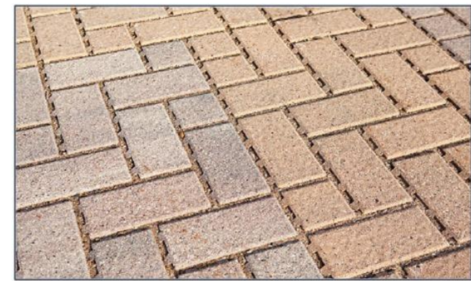
Porous + Permeable Pavements
